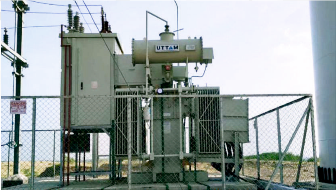
3.0 MVA Inverter Duty Transformer 33/0.690kV for Wind Application
