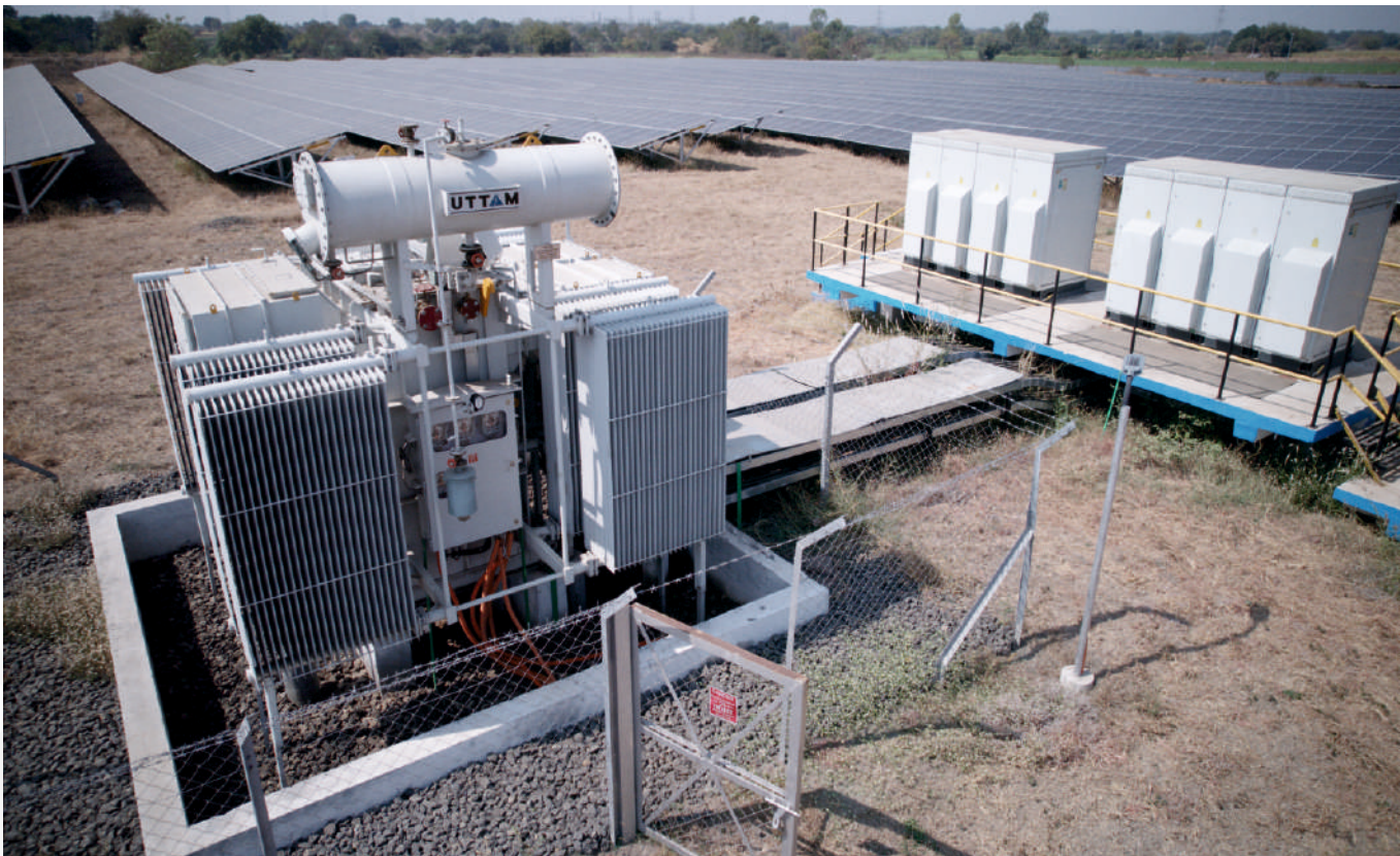
7.8 MVA Inverter Duty Transformer 0.660-0.660/33kV for Solar application
